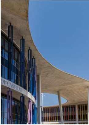
Zaragoza 2008 – National Pavilions building.
