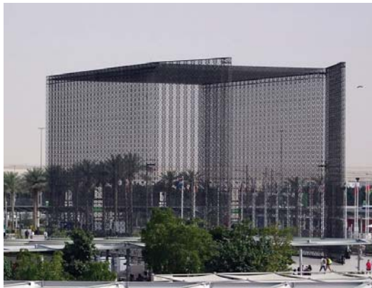
Mobility district entry gate.
